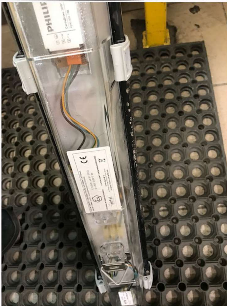
Fig. 3. Interior of the fixture after the climate tests.
