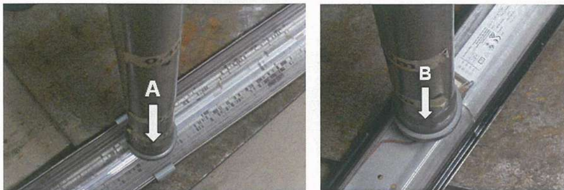
Fig. 4. Spot of swingle impact in the fixture enclosure.
