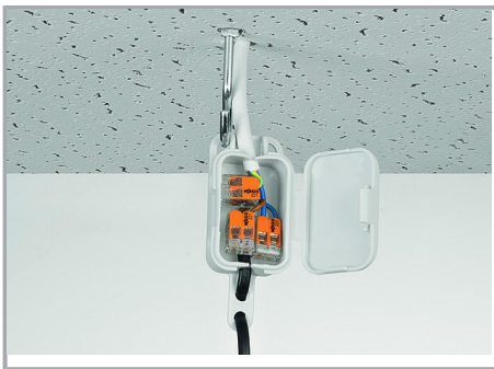
Pendant light connection in a suspended ceiling
